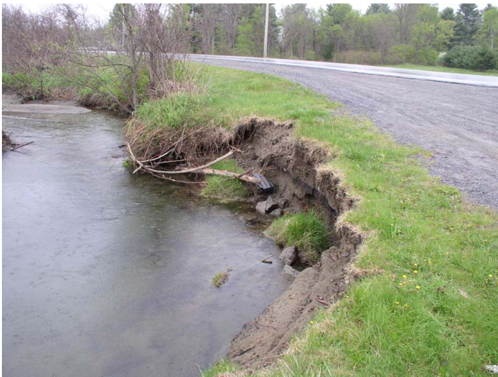
Trout Brook along the Rte. 10 pull-off area just north of Balch field has meandered on this reach causing severe erosion. It is a safety concern for the highway.
