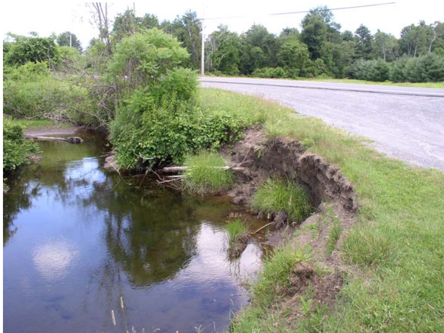
The streambank erosion on Trout Brook has not worsened during the summer rains, but vegetation has not stabilized the bank, particularly where it is undercut.
