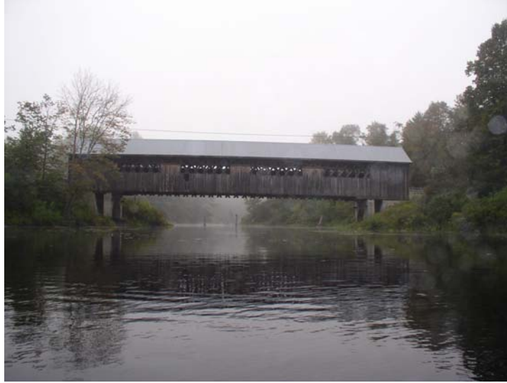
Edgell Covered Bridge on Clay Brook at the confluence with the Connecticut River. Built in 1885, it is 132 feet long.
