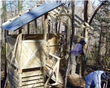
Photo from the web of a moldering privy from the outside to show the project's potential size and complexity. This was taken on the Appalachian Trial.
