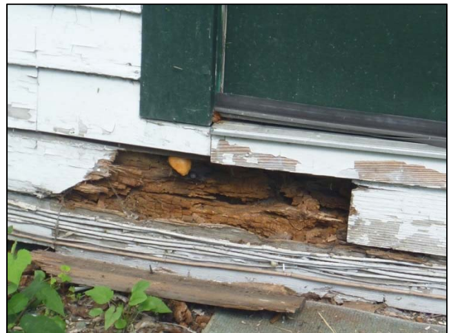
Above: Decaying wood on the exterior of the Orford Town Office Building.
