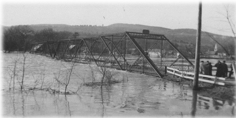
North Thetford Bridge, flood March, 1936
