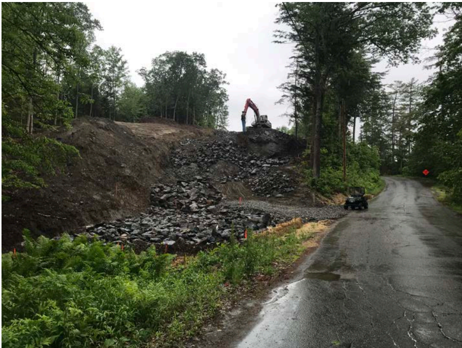
PHOTO 4 – Ledge removal at north end of the project.
