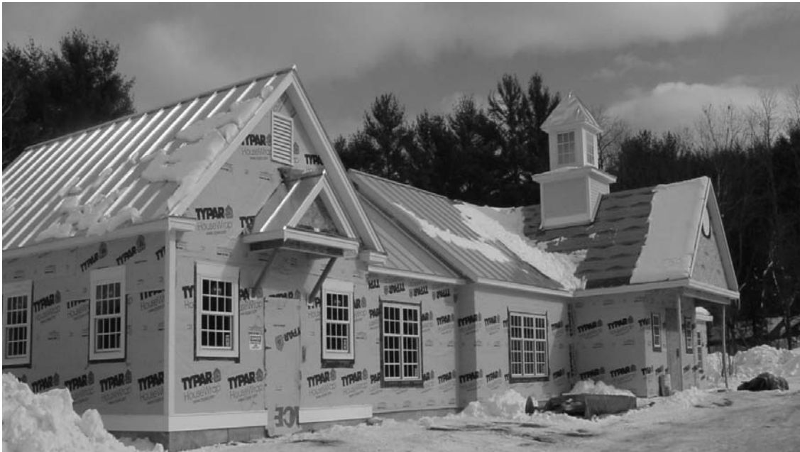
NEW MUNICIPAL SERVICES BUILDING
